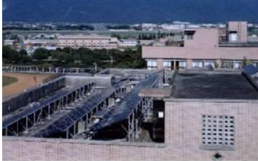
Fig. 4. Solar hot-water systems in Hualien County Hualien Academy for 115 students (Metallic collector installation area: 77 square meters)
