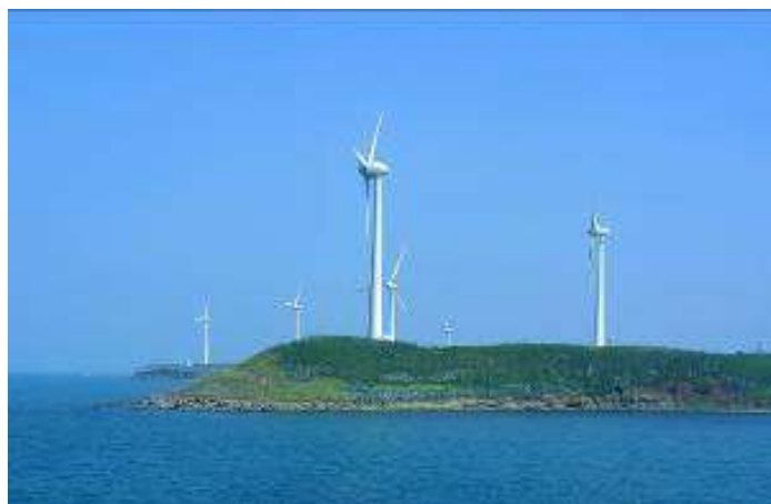
Fig. 10. Taiwan Power Company Penghu wind power (Installed capacity: 600kW x 8)
