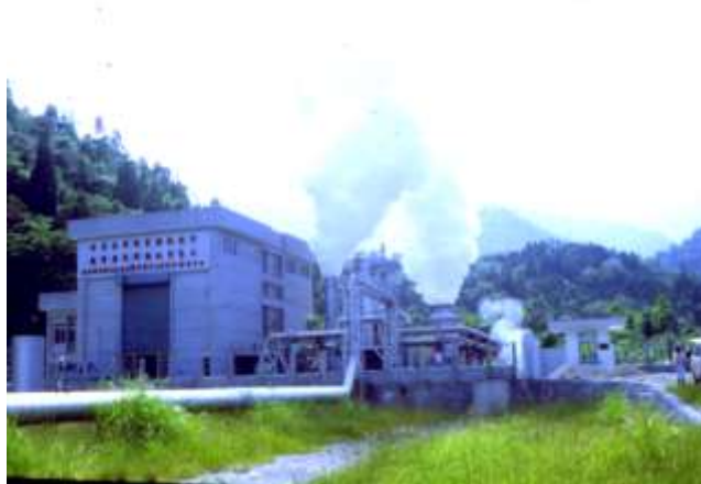
Fig. 15. Chinsuei geothermal energy project, 3MW, single flash-steam
